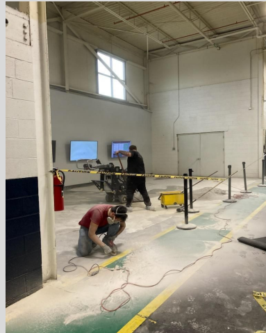
Victor Esquivel and Eric Haskins resurfacing the KPI floor
